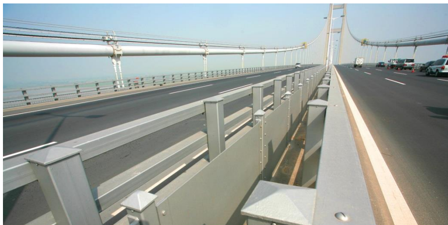
Fig. 4 Central stabilizer mounted on Runyang Bridge
