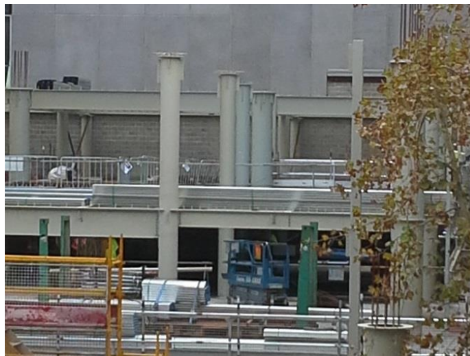
Fig. 4 Spiral welded steel tubes, Perth Tower, Australia
