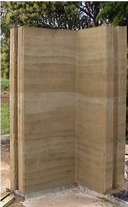
Figure 2 - Example of conventional rammed earth wall (Piripono Kura Construction Trial 2004)
