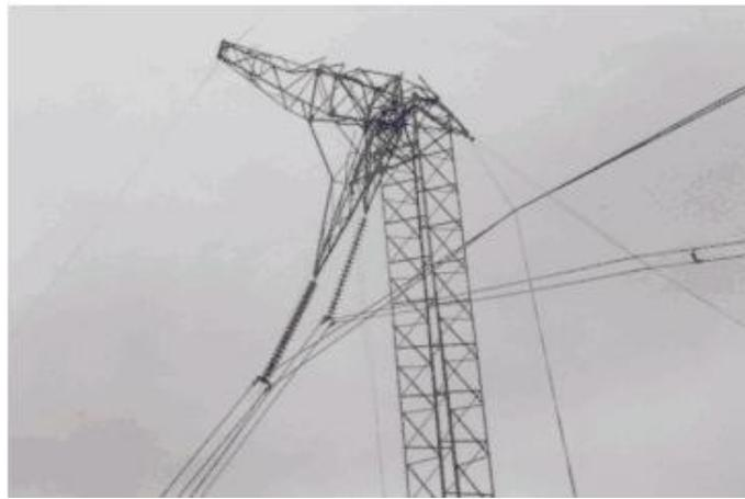
Fig. 12 Field evidence of lattice tower failure at cross-arms (Manitoba Hydro, 1999)
