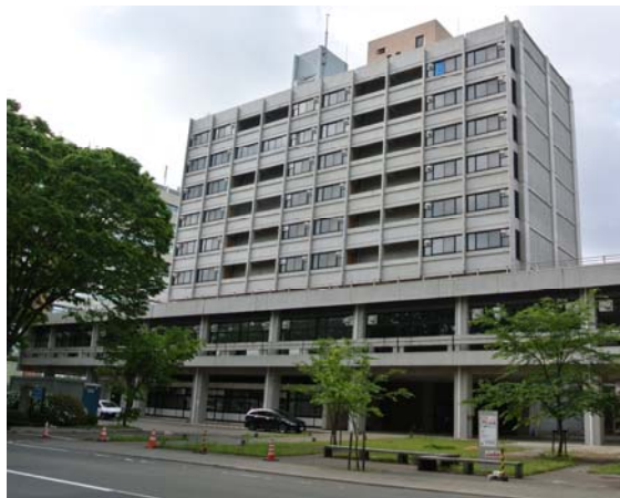
Figure 1: Former research building of Department of Civil Engineering and Architecture, Tohoku University
