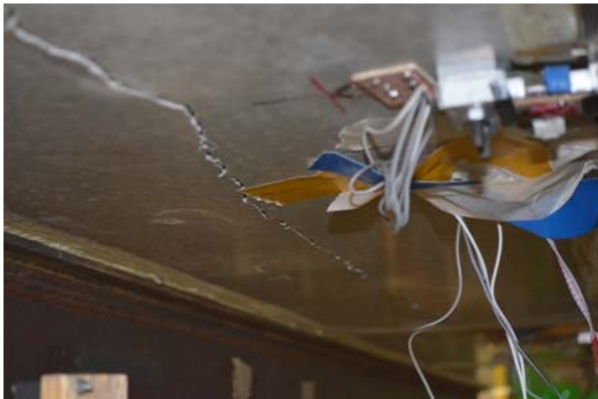
Fig.6 Observed crack in the testing
