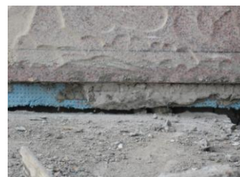
Fig. 2 Close-up views of a positioned LRB and horizontal isolation seam
