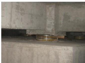
Fig. 2 Close-up views of a positioned LRB and horizontal isolation seam
