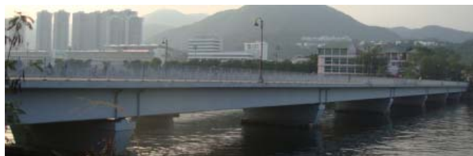
Figure 2 Overall view of Footbridge NF276
