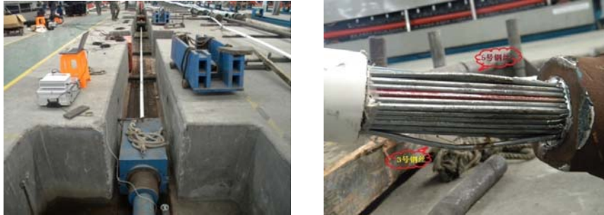
Fig. 6 Cable stretch equipment and breakage wires
