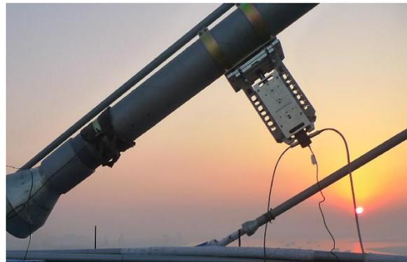
Fig.2 Vibrator attached to the cable
