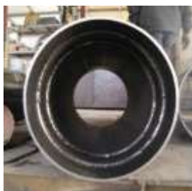
Fig. 5. Shear keys on pile
