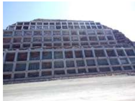
Fig.2 after the supporting
