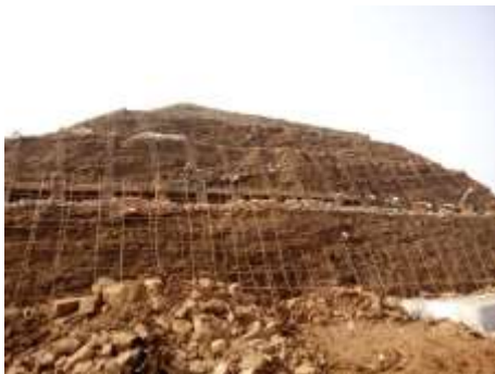
Fig.1 before the supporting
