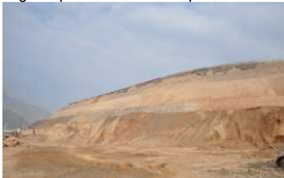
Fig. 4 Cut slope on site
