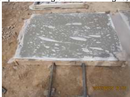
Fig. 8 Anchor plate casting
