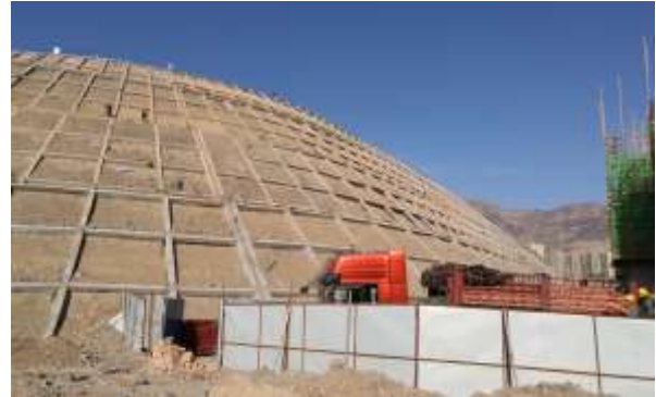
Fig. 11 Overall completion elevation of slope
