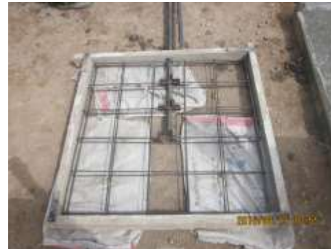
Fig. 7 Anchor plate reinforcement
