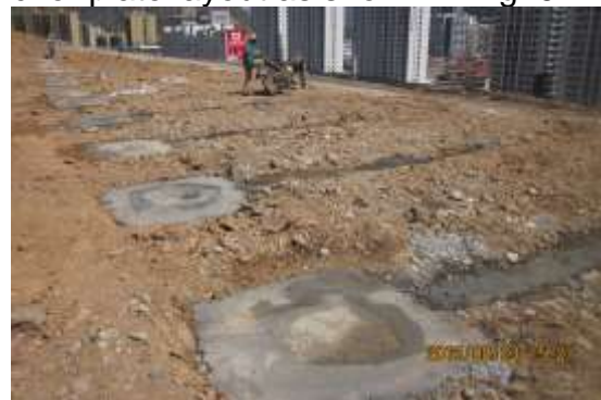
Fig. 9 Anchor plate layout
