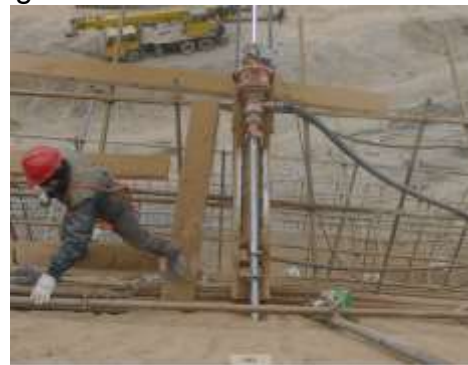
Fig. 5 Drill hole of anchor
