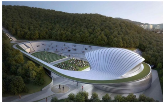
Fig. 1 Membrane structure of Gwangju Sajik Park
