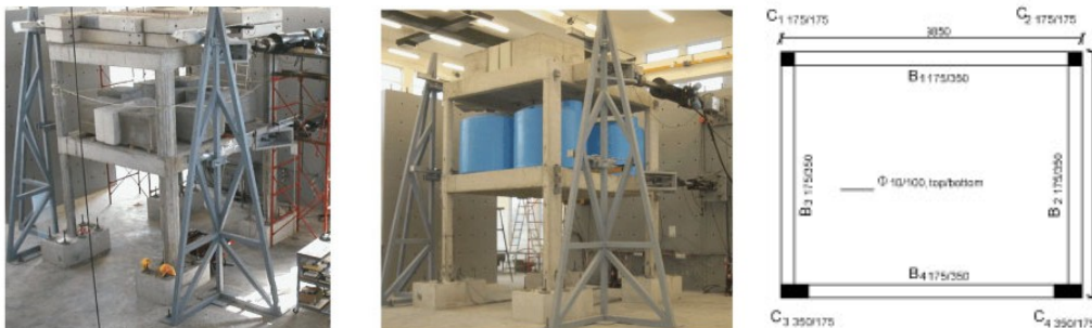
Fig. 16 1-bay, 2-story reinforced concrete building in Bousias et al 2007
