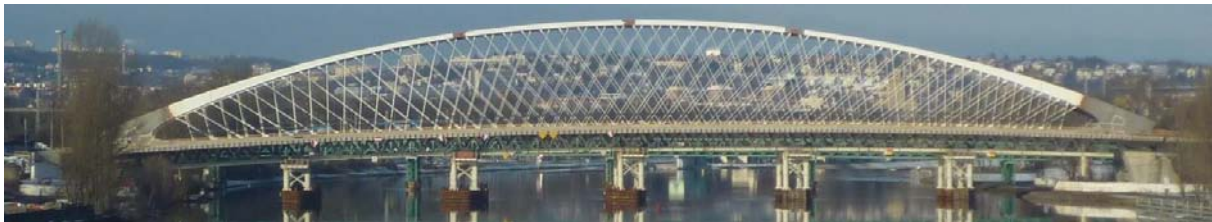
Fig.10 View of the structure with hangers
