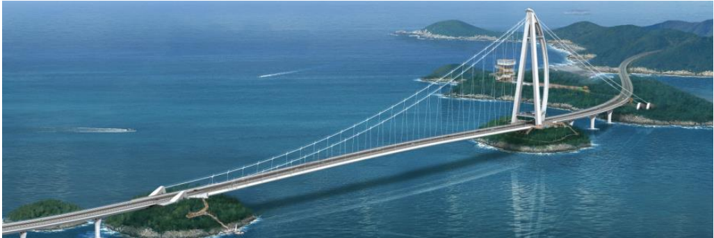
Fig. 2 Aerial view of Dandeung bridge
