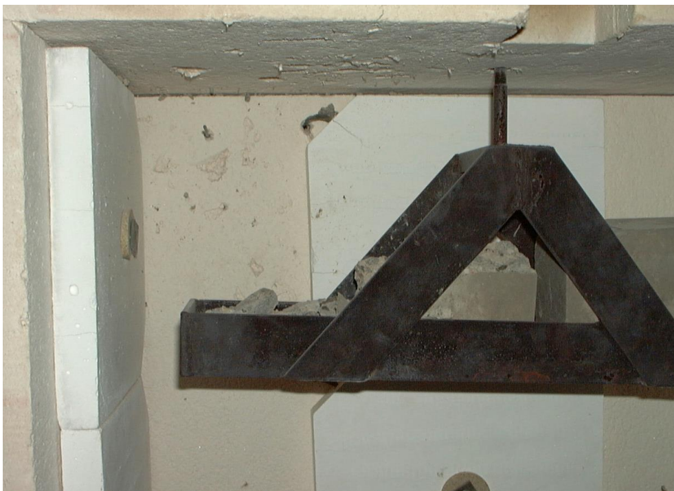
Fig. 8 Partial spalling of a concrete prism in the cradle for 10°C/min
