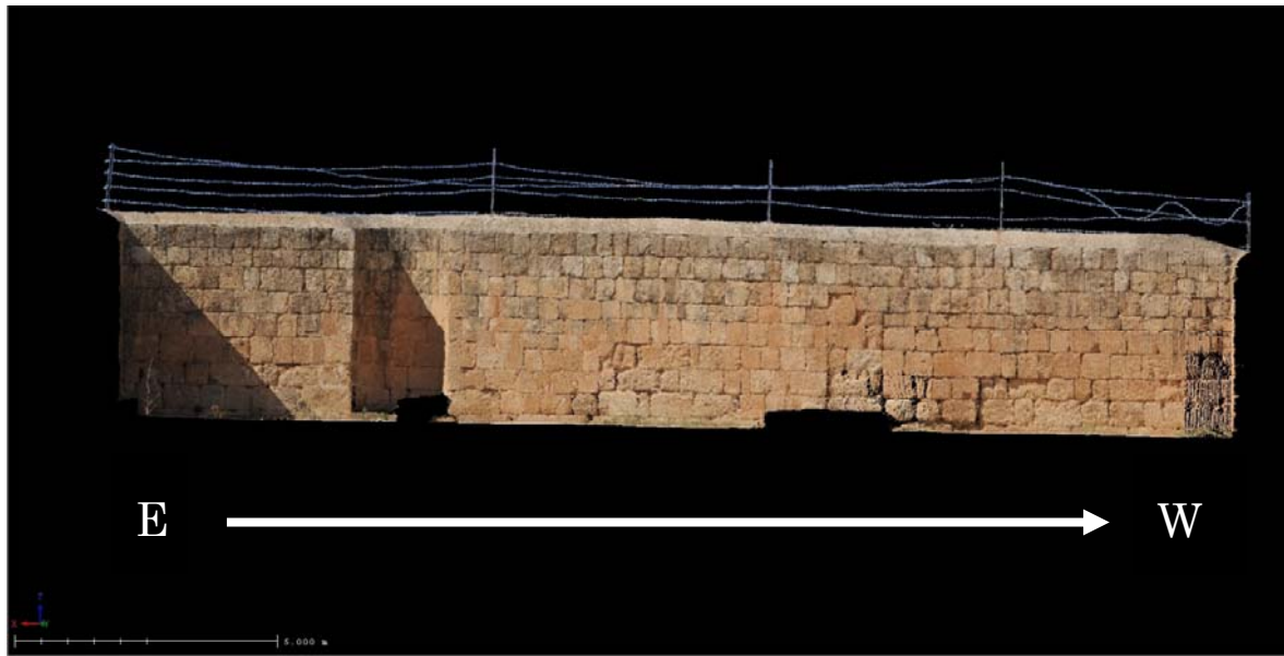
Fig. 1 Inclination of the ground towards the west (wall between Sts. Cosmas and St. John the Baptist)
