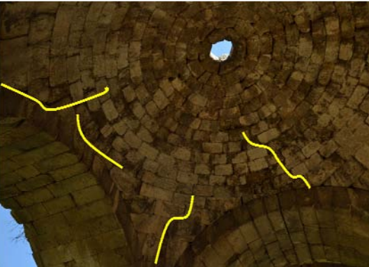
Fig. 8 Inner surface of the dome
