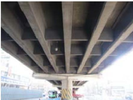
Figure 2. PCI Girder Bridge
