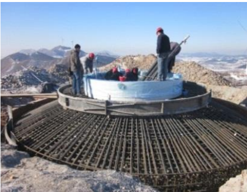
Fig. 1 The construction site of the RC foundation
