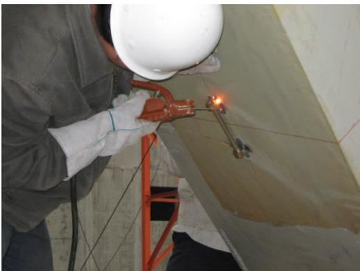
Fig. 5 Installation of sensors
