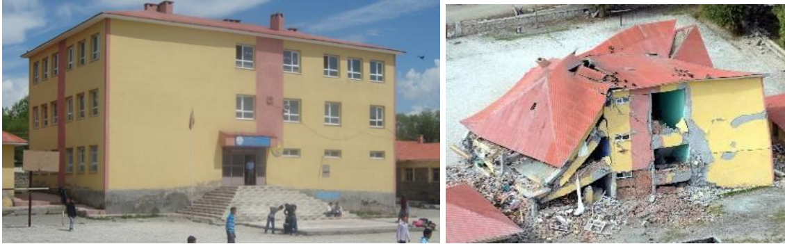
Fig. 14 Failure of a symmetrical school building
