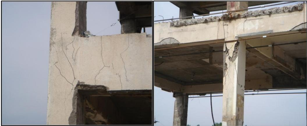
Fig.7 Crack of exterior beam-column joint Fig.8 Central column failure
