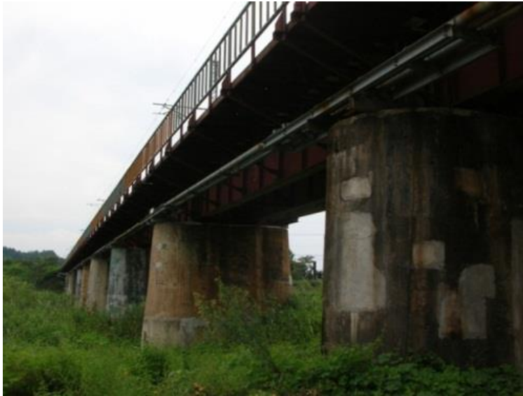
Figure 1 Typical TOSPG Bridges
