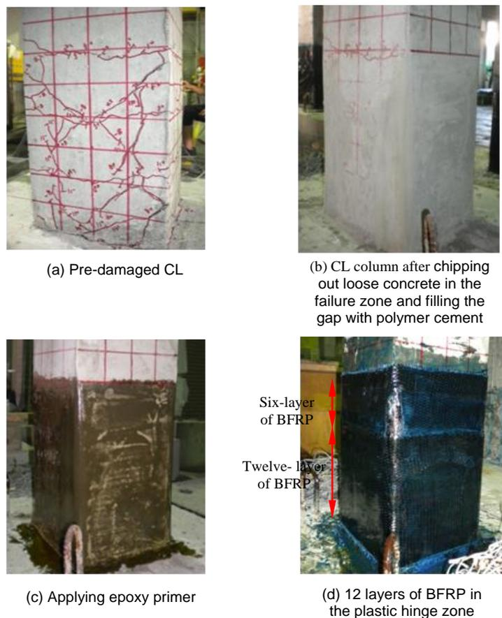
Fig.5 - Repairing procedure of CL column using polymer cement and BFRP Jacket
