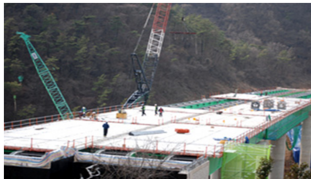
Fig. 1 Rapid construction of precast concrete bridge decks
