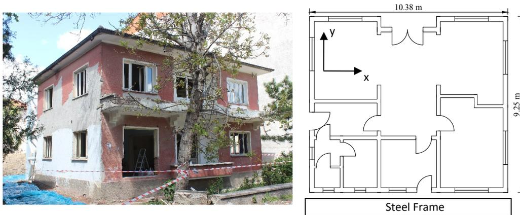
**Figure 8.** Photo and plan view of the second test structure
