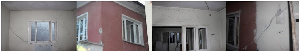
**Figure 17.** Different cracks observed during one-way cyclic test
