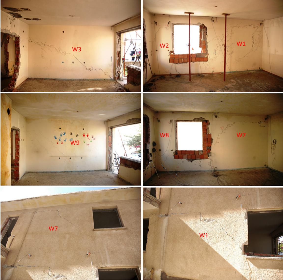
**Figure 15.** Observed Wall Damages
