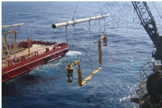
Fig. 2 The installation of subsea jumper
