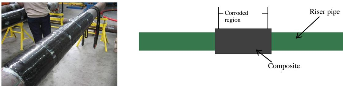
Fig.1 Riser repair(a)outside view,(b)schematic diagram
