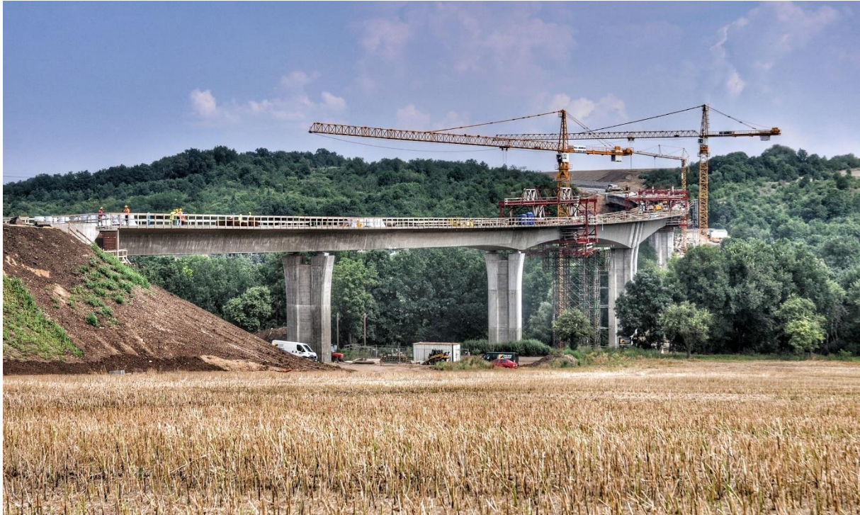
Fig. 3 Overall view of the bridge during construction process
