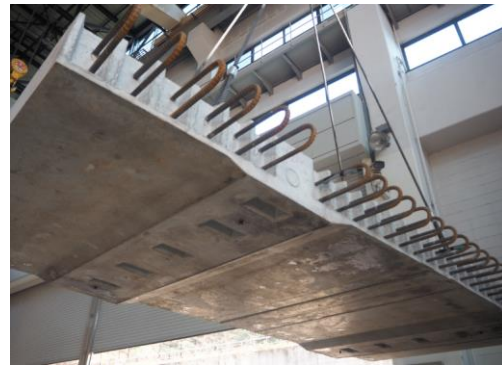
Fig. 2 Precast deck module with ribbed loop joints
