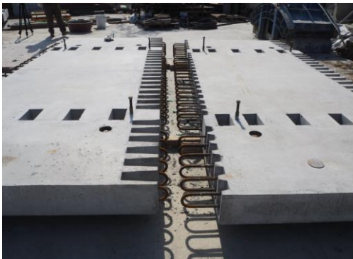
Fig. 3 Connection between precast deck modules
