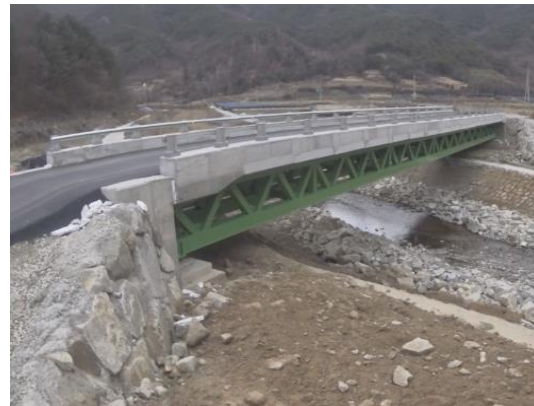
(b) Road bridge
