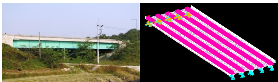
(a) A steel plate girder bridge
