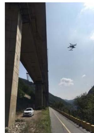
Fig. 5 Inspection using UAV
