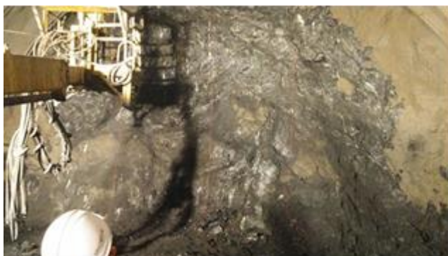
Figure 3. Status of tunnel face
