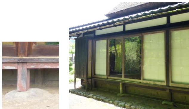
Photo 7. Post erected on a foundation stone
