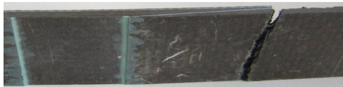
Fig. 12 Damage modes of tapered flush joints
