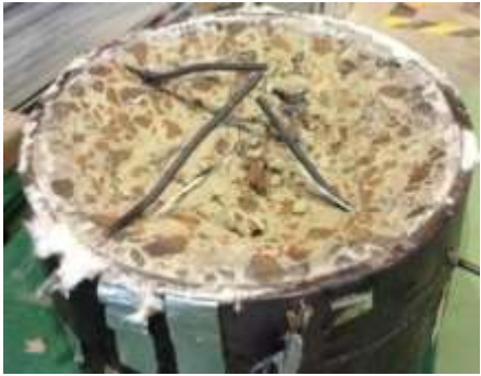
Fig. 10 Spalling after heating test
