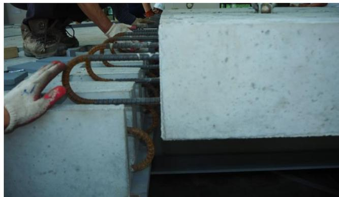
Fig. 3 Precast deck system allowing vertical installation
