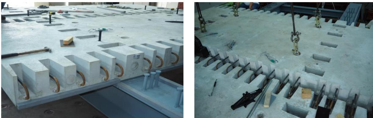
Fig. 2 Connection of precast deck with ribbed loop reinforcement
