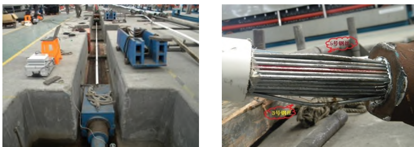
Fig. 6 Cable stretch equipment and breakage wires
