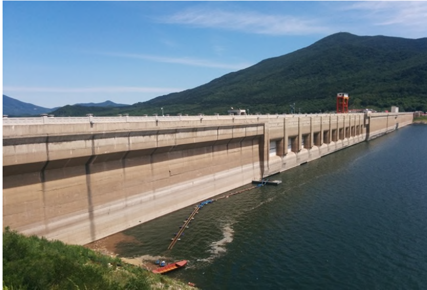
Fig. 3 Upper stream view of the Fengman dam
