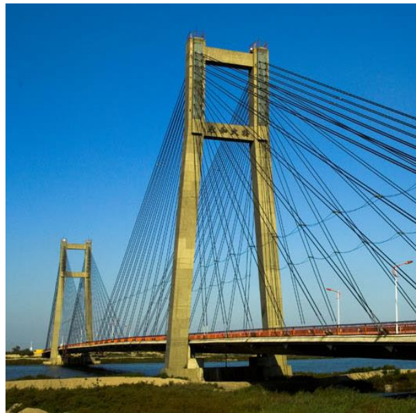
Fig. 1 Overview of the cable-stayed bridge
