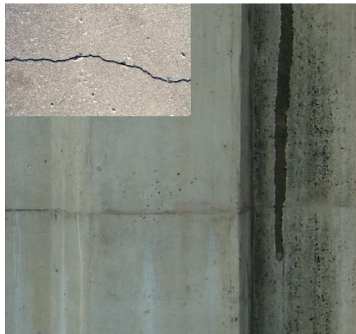
Fig. 2 An example of hard negative images merged with a clean crack image.
