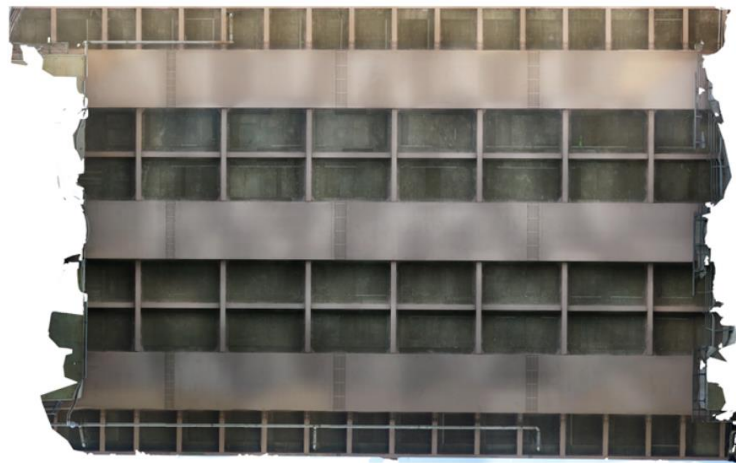
Fig. 4 Slab Orthomosaic Image of Tancheon Overpass
