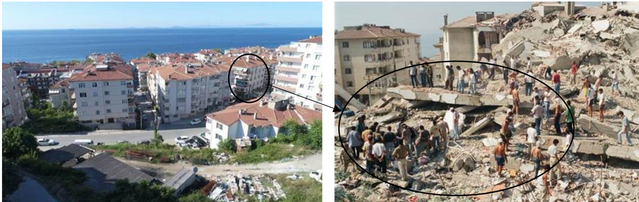
Fig. 1 Before and b) after views of collapsed RC structure.
