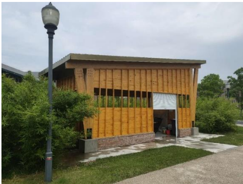
Fig. 1 Waste treatment building on Haining Campus of ZJU
