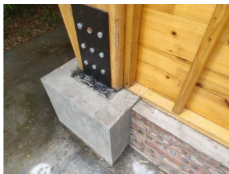
Fig. 3 Recycled concrete used in Recycling center
