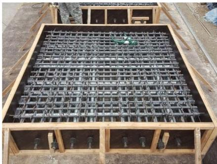
(a) Placement of rebar and ducts
