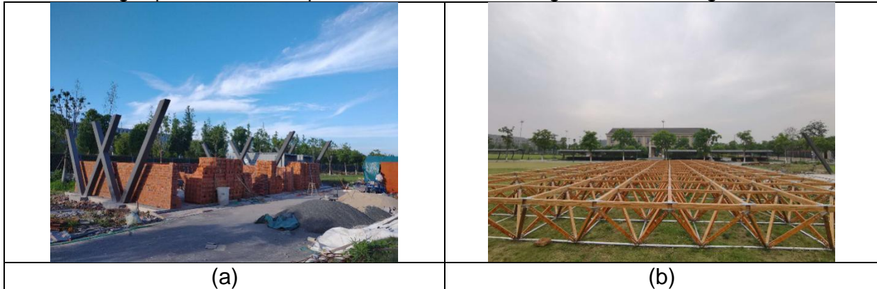
Fig.8 Construction update: (a) steel frame; (b) bamboo-steel truss assembling on ground.
