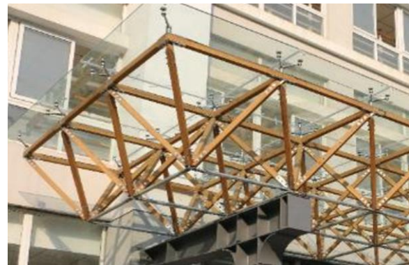
Fig.4 Bamboo-steel truss 1
