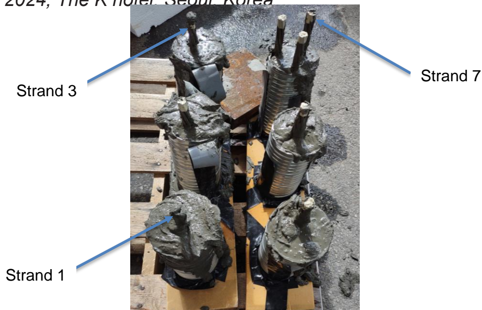
Fig. 3 Short tendons being grouted
