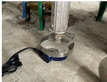
Fig. 1 Measurement of shore load using load cell
